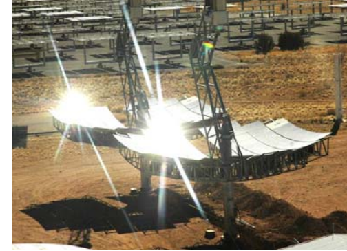
National Solar Thermal Test Facility (SNL, NM)
