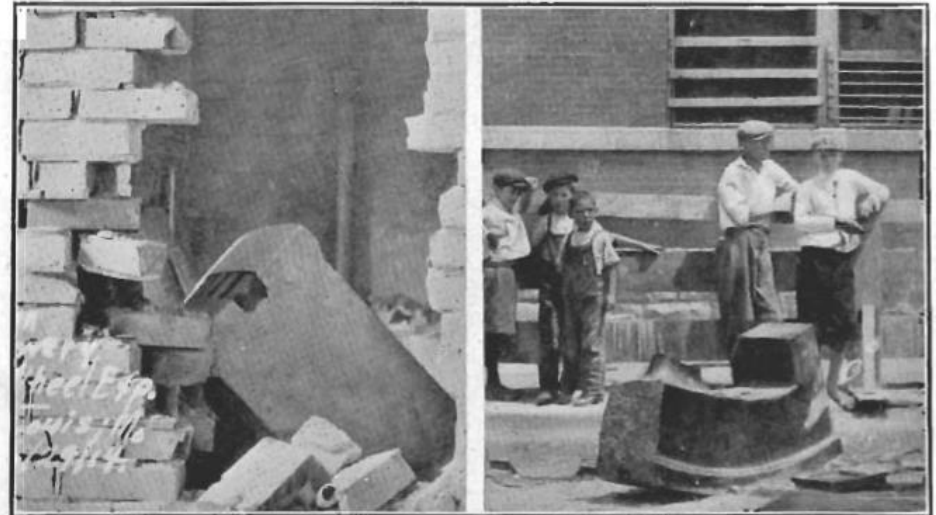
FLY-WHEEL EXPLOSION UNION BREWING CO., ST. LOUIS, MO., 40,000- POUND WHEEL ON ICE MACHINE RUNNING NORMALLY AT ONLY 50 R.P.M. MACHINE RACED AND BURST WHEEL BY CEN- TRIFUGAL FORCE, HURLING 8,000-POUND CHUNKS GREAT DISTANCES. RIM SECTION WAS 13"x16", TO BREAK WHICH REQUIRED 4,000,000 POUNDS. LOSS $13,423. WHEEL INSURED.
